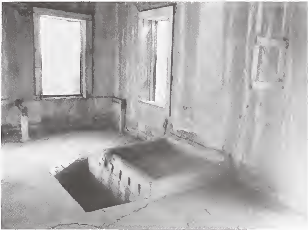
Figure 18. Interior of assay office, showing concrete tub features likely used to process gold. Photo by Richard W. and Florence B. Lord.
